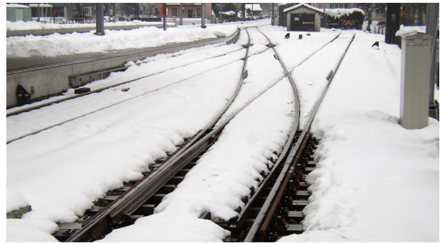
Fig. 12 Gas switch heating (Image by FabiBerg/Wikimedia Commons distributed under CC BY-SA 3.0 license)
